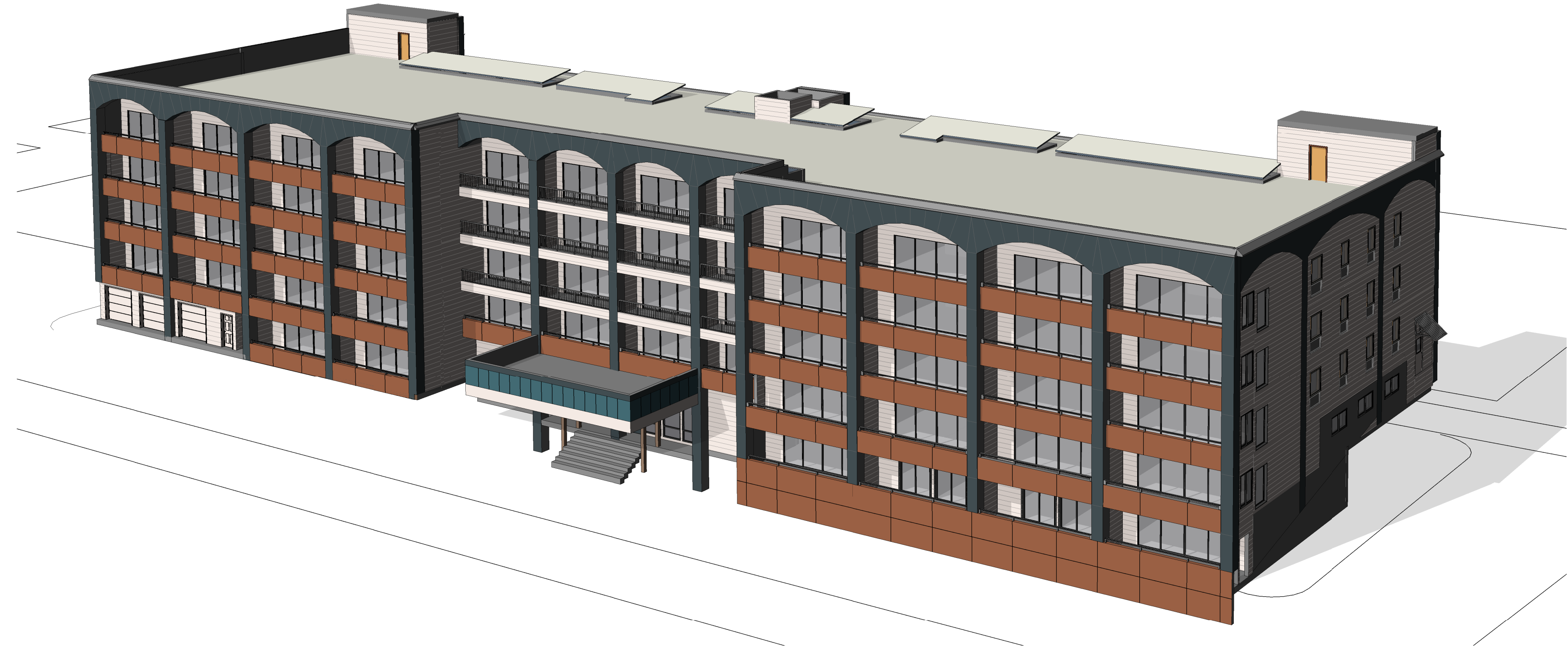
① AERIAL VIEW FROM SOUTHEAST
